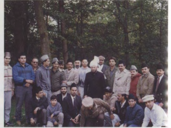
Ground Breaking - Washington Mosque
