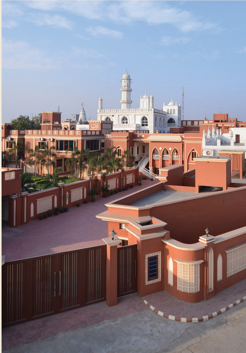
A view of Qadian.
