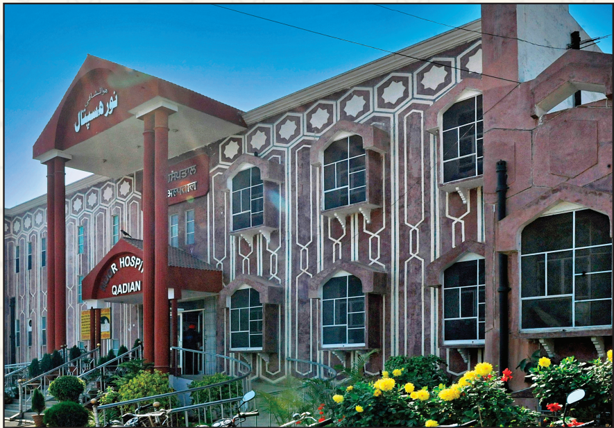
Noor Hospital (new building)
